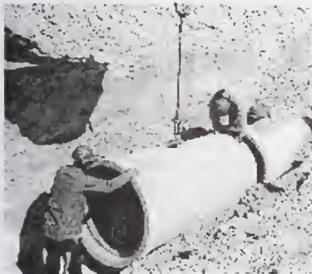
a) Laying Pipe Traditionally
